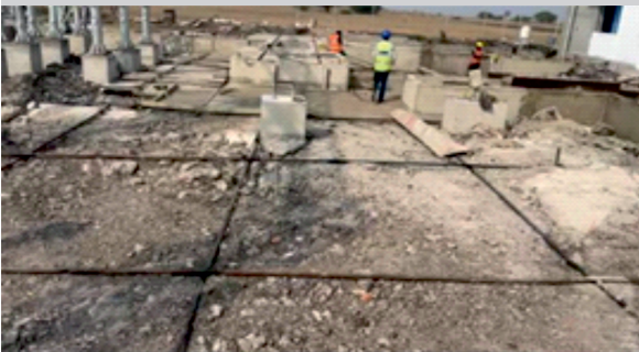
SWITCHYARD MESS EARTHING WITH 400 MM ROD
