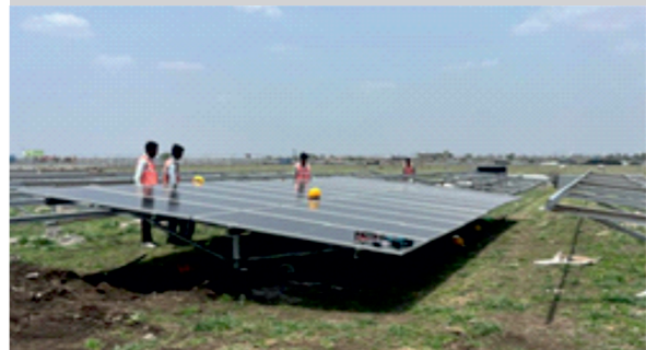
SOLAR BLOCK INSTALLATION
