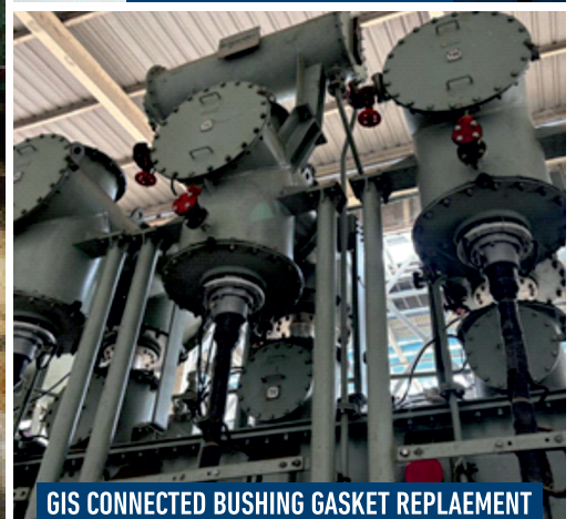
INDIAN RAILWAY- 220KV TRANSFORMER BUSHING SUPPLY & INSTALLATION
